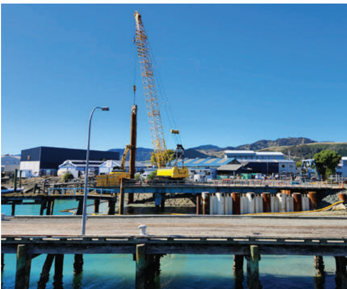
AIMEX Nelson Port Slipway
