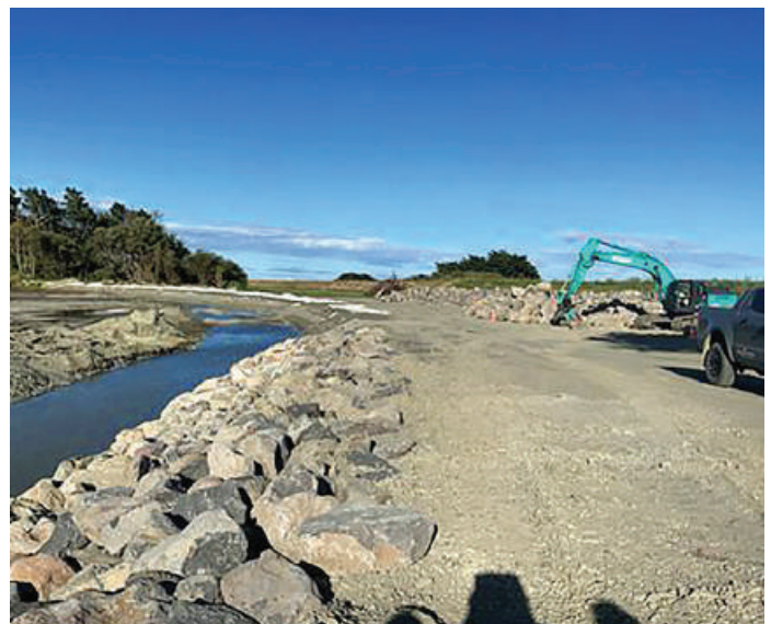
Rangitikei River Enhancement Te Hou Rock lining
