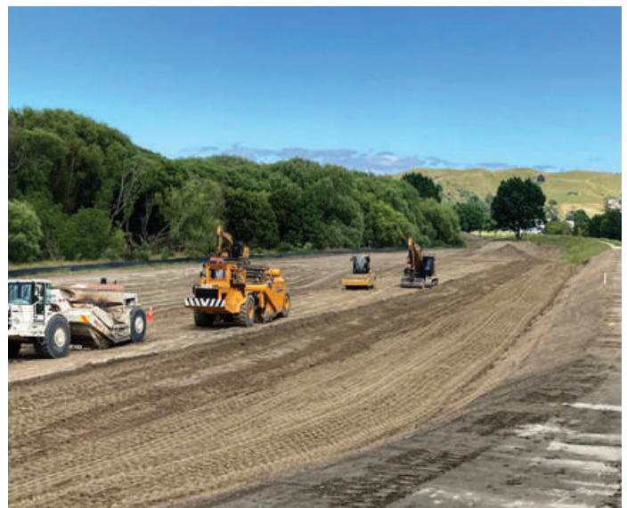
Heretaunga Plains Flood Control Protection
