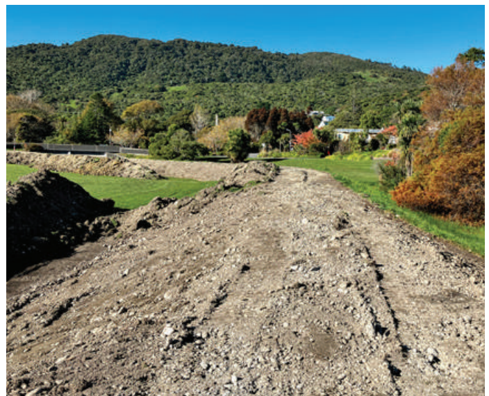
Grey Floodwall Protection
