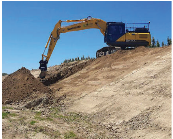
Waipaoa River Flood Control Scheme
