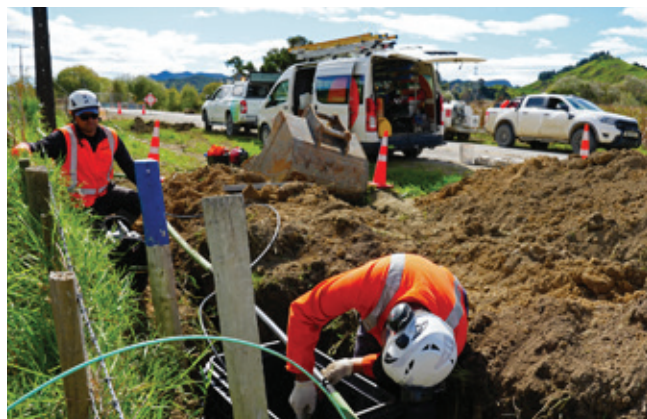
Chorus Hikuwai Bridge rebuild 2023
